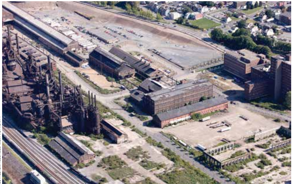
The site before redevelopment.
